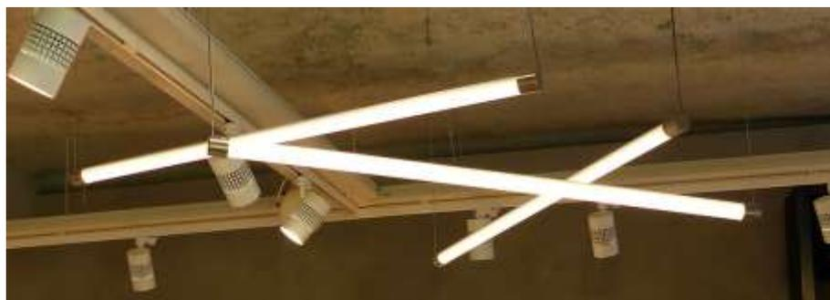
Suspensions Led style néon, tube opaque, source 1000lm / ml
